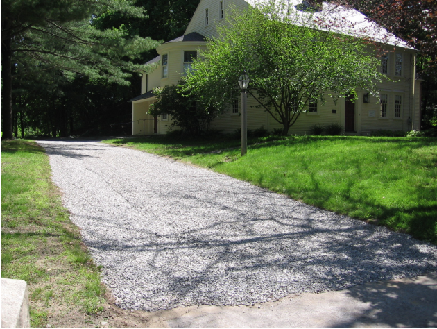
Entrance from 27/126 intersection
