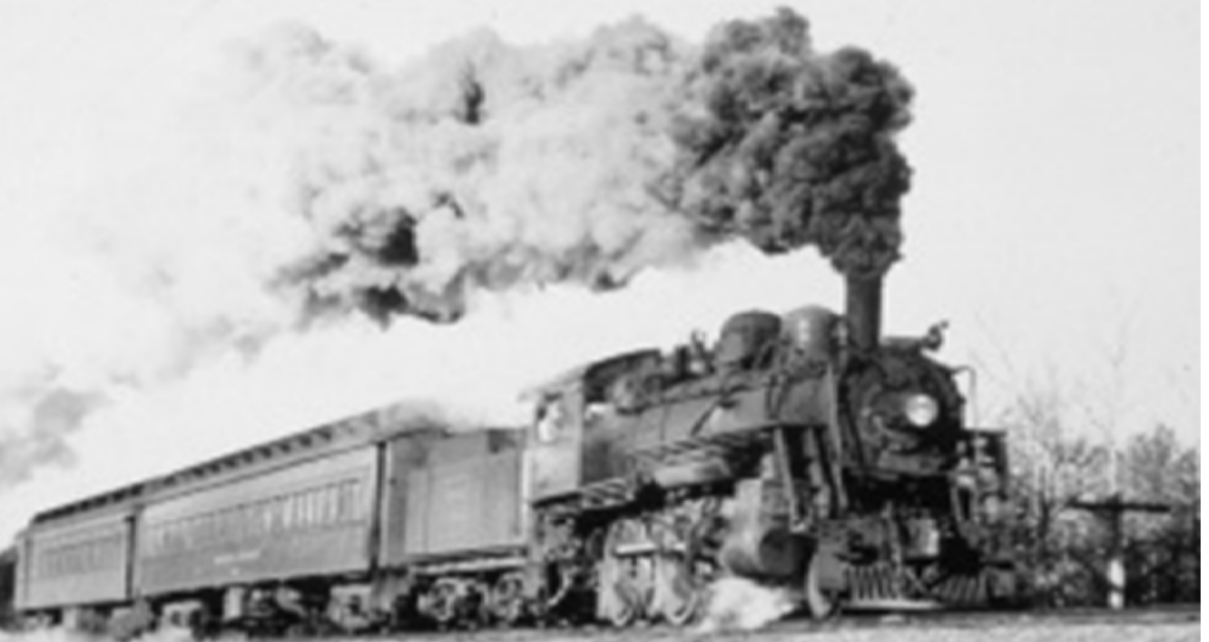
Mogul 1496 hustles train 3106 into Wayland's Tower Hill Station in 1956
