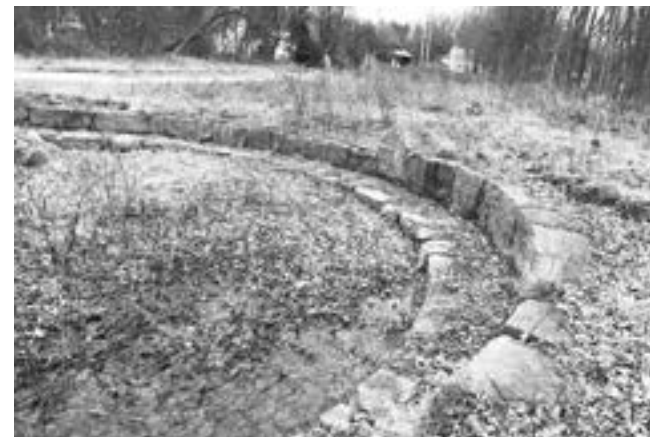
The turntable had two granite-block rings. The inner, lower ring had a circular rail, on which sat a large frame with flanged wheels. Everything was so well balanced that the frame, with a railroad car or locomotive on it, could be rotated by human power. (Photo by Paul Penfield Jr.)
