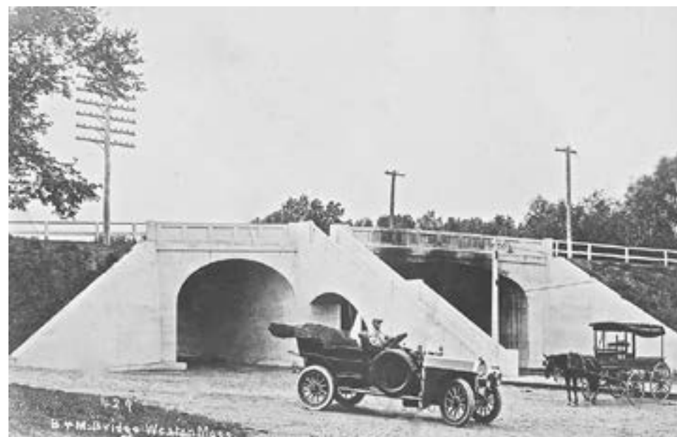
This reinforced concrete bridge was constructed in 1911-12 to eliminate the grade crossing at Church Street. The station was relocated at that time. The smaller arch allowed wagons to pass between the relocated station and the freight spur track, which remained in its original location west of Church Street. The bridge on Concord Road was constructed at the same time. Petitions were made to eliminate grade crossings on the Fitchburg line but that work was never carried out. (Weston Historical Society postcard, c. 1912)
