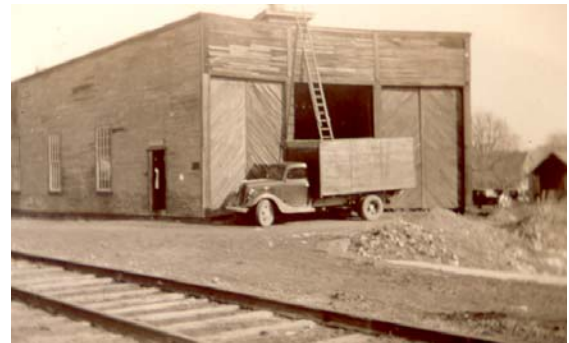
Figure 14. Historic view of engine house, in 1938, (photograph by Henry Gibson, courtesy Beverly Historical Society).
