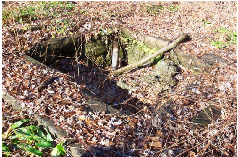
Figure 16. The foundation remains of the water tank, (HWA, 2004).
