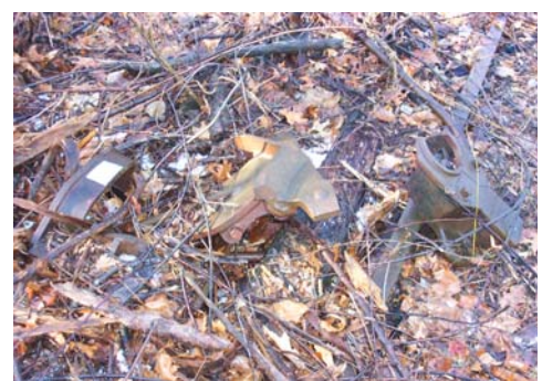
Figure 10. Broken derail mechanism (HWA, 2004).
