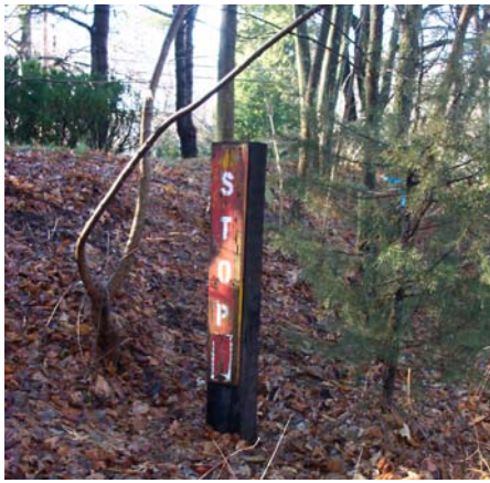
Figure 11. Wood stop post, (HWA, 2004).
