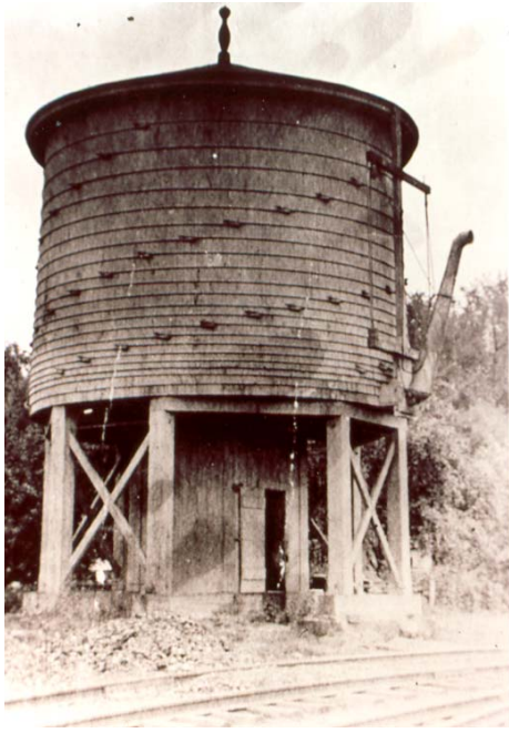
Figure 15. The water tank in 1915, (courtesy Walker Transportation Collection, Beverly Historical Society).
