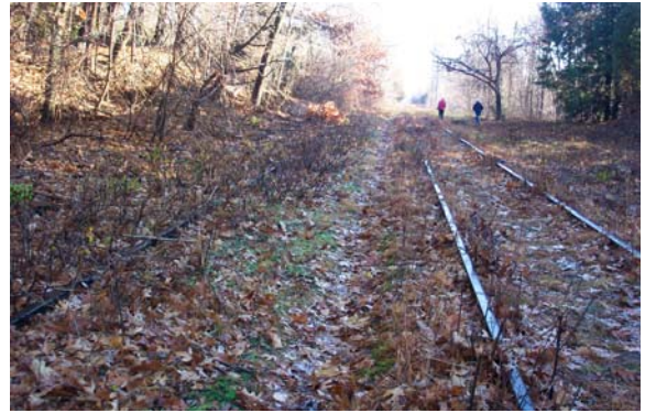
Figure 7. Main line and siding, east of the freight house (HWA, 2004).
