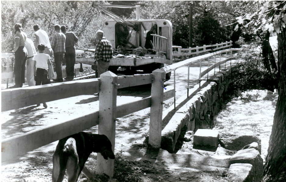
"Water rushing under old bridge on Stonebridge Road Sept. 12, 1953" Viewed from Wayland facing Framingham. From the Wayland Historical Society's collection.
